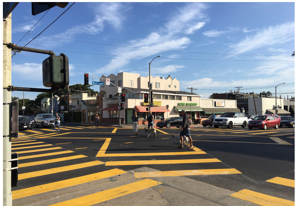
Scramble crosswalk at Pacific Ave. and Washington Blvd.
