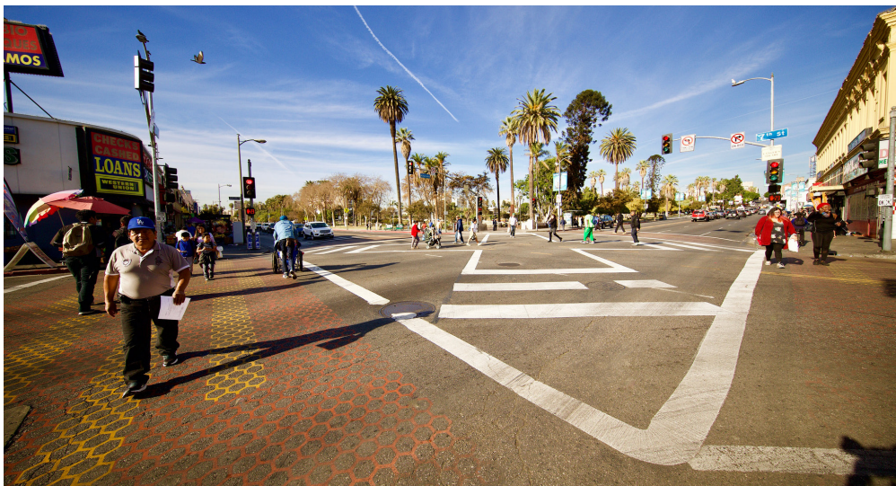
New scramble crosswalk at the intersection of Alvarado St. and 7th St.
